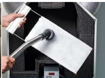
Reinigen wtw-filters
